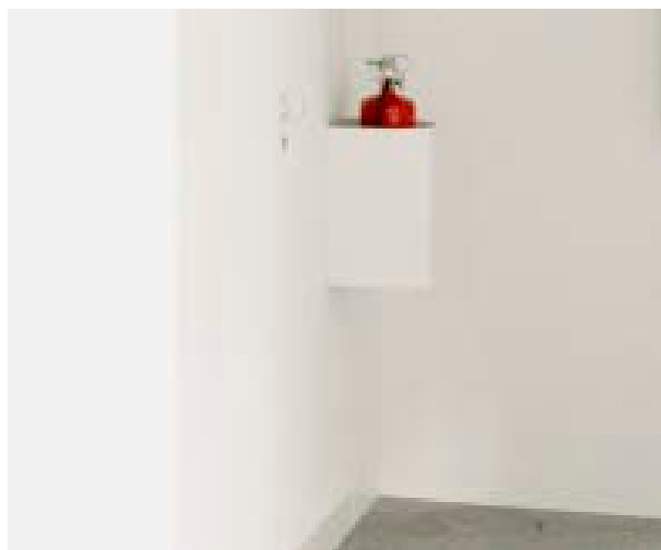
Relocated fire extinguisher on outer wall of a closet
